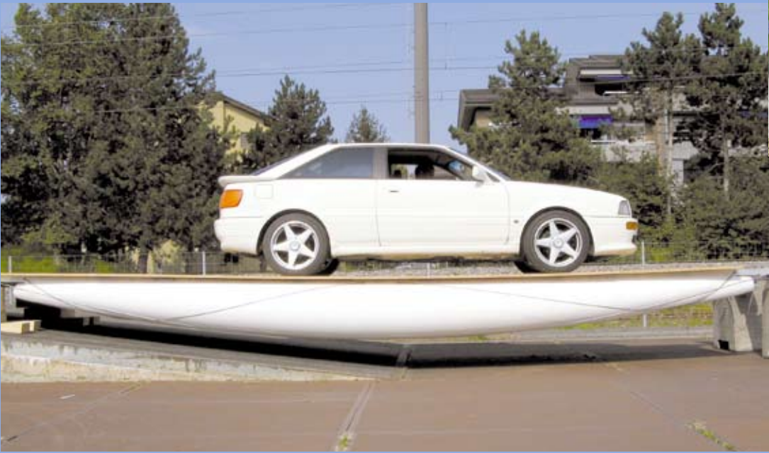
This demonstration bridge with an eight-metre span easily holds large loads such as a 1.5-tonne automobile.
