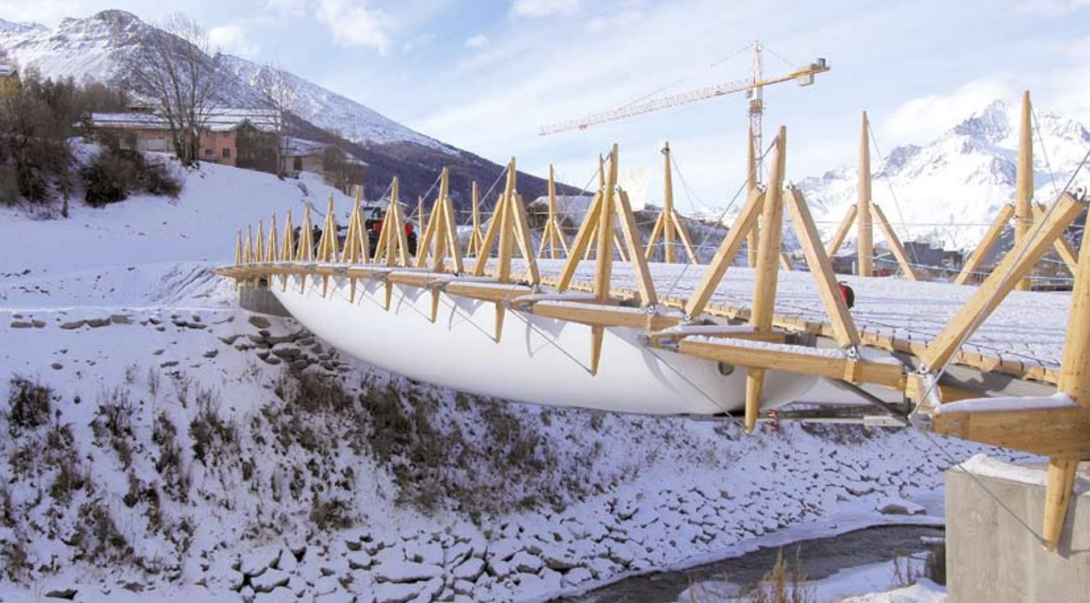
52-metre span: This ski bridge in the French Alps uses the pneumatic supporting structure Tensairity. PVC-coated fabric filled with air plays an important role in this process.
