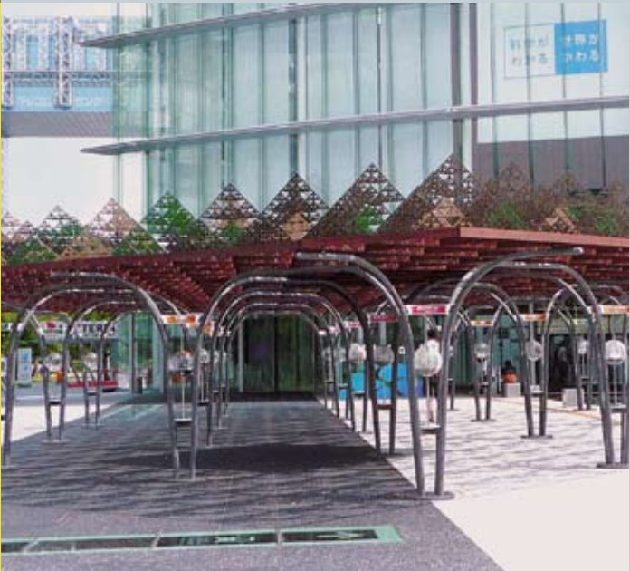
Re-creating the natural shape of the leaf: This fractal triangle continuously retains little heat and is cooled down by means of air circulation.
