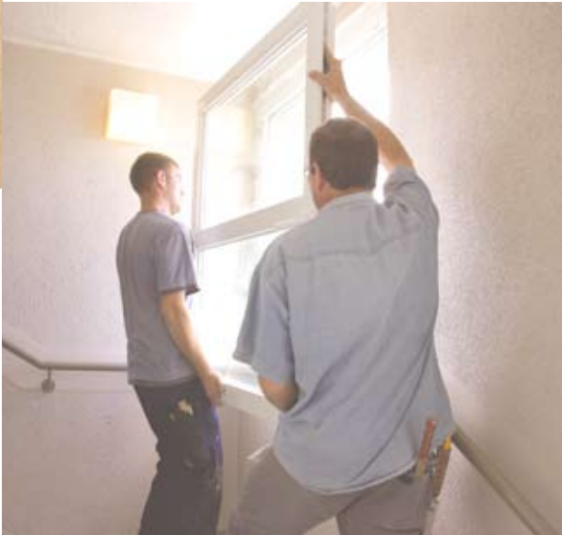
An integral part of the energy-saving modernisation project in the Märkisches Viertel is the replacement of old windows with modern energy-saving systems.
